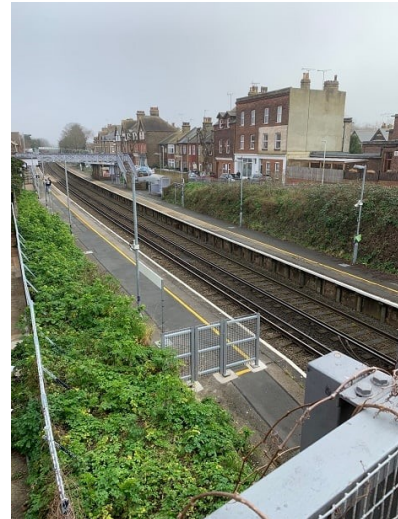
Figure 19-1 Westgate Railway Station
